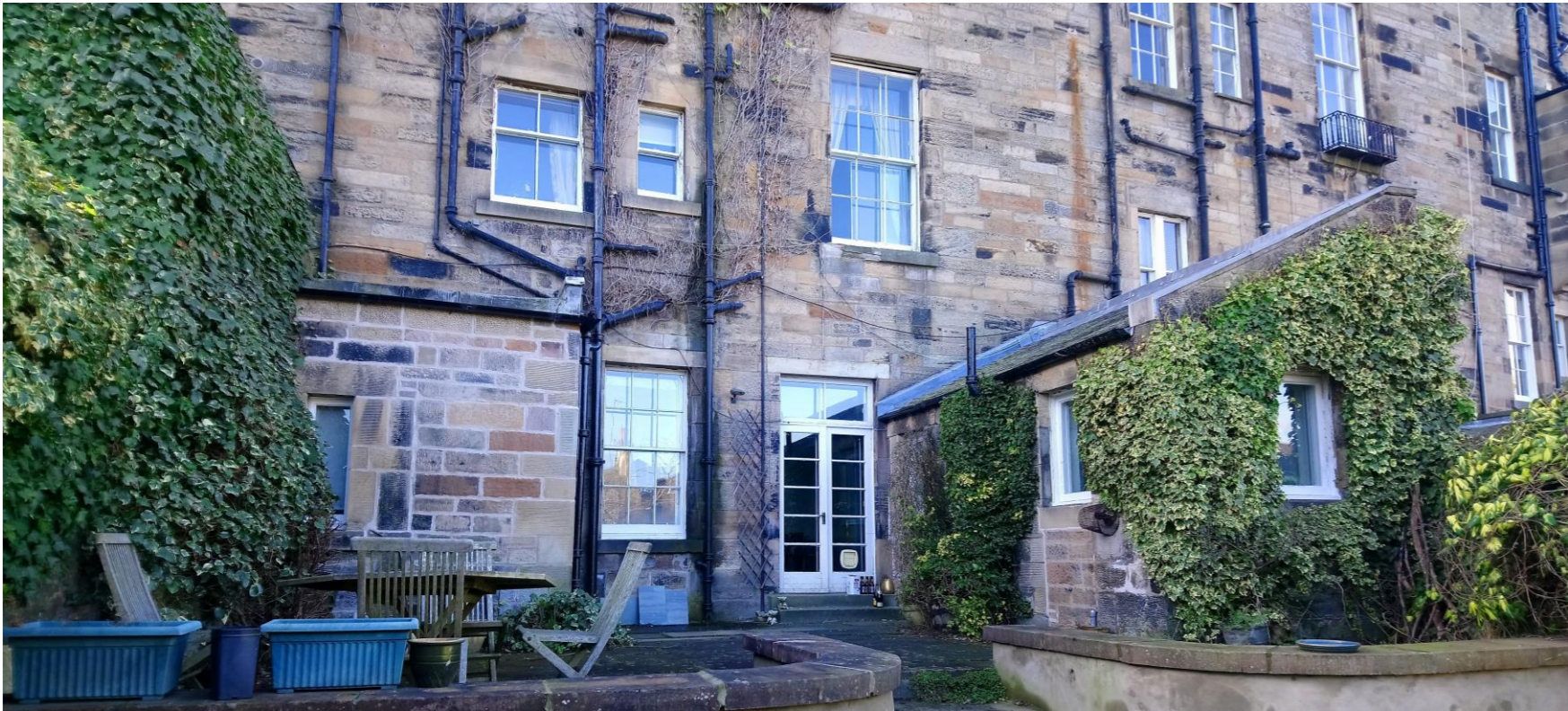
View 1 External view from lower garden
